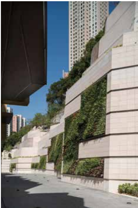
Blue Pool Road Residential Development: Living Walls integrated with Retaining Walls
