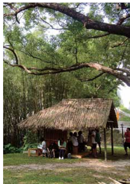
The hut is oriented to capture the lakeside view of the zigzag bridge framed by arching bamboo blades.
