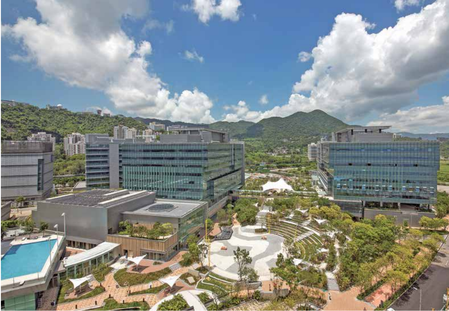
View from courtyard and lotus pond
