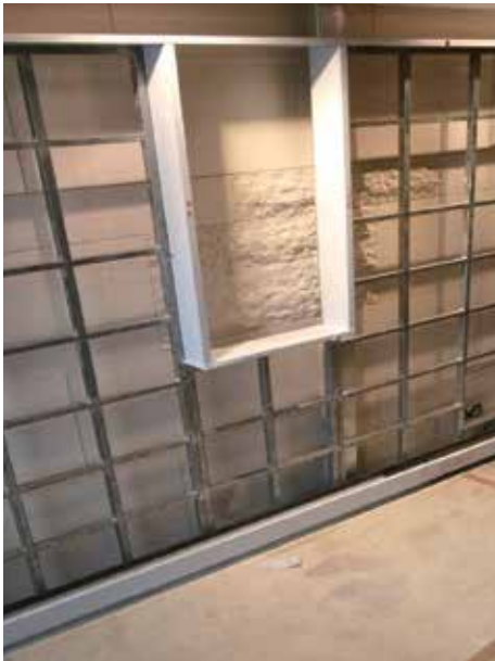
RLP Office: Installation of Living Wall
