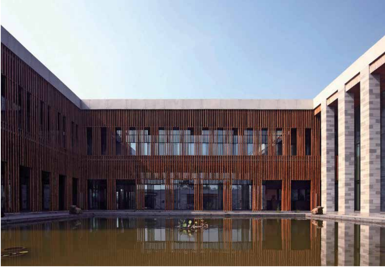
View from courtyard and lotus pond
