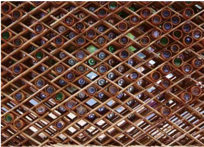
Inscribed scrolls are wrapped around recycled plastic water bottles of different colours. The layers of standard folding fence are carefully angled to create suitably-sized slots for the rolled-up scrolls.
