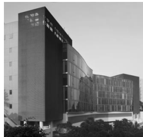
2006 A Purpose Designed Building for Centralised Science Laboratories, The Chinese University of Hong Kong 香港中文大學實驗室專門大樓 HKIA Merit Award 香港建築師學會優異獎
