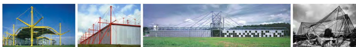
Figure E3.4: Cable Stayed Structures. Examples]
