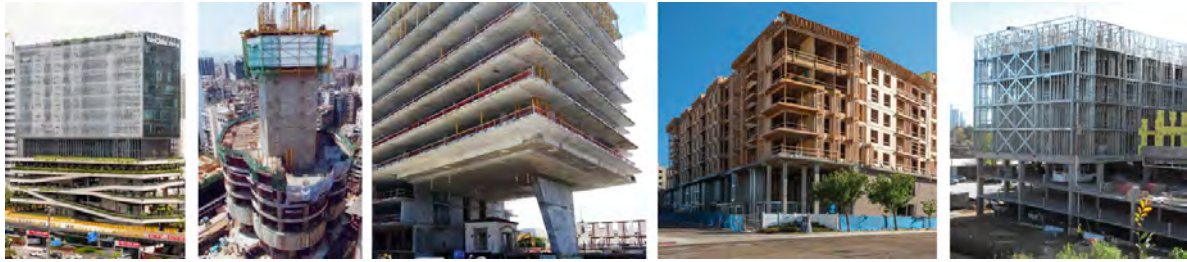
Figure F1.15 Transfer Plate structures. Examples.
