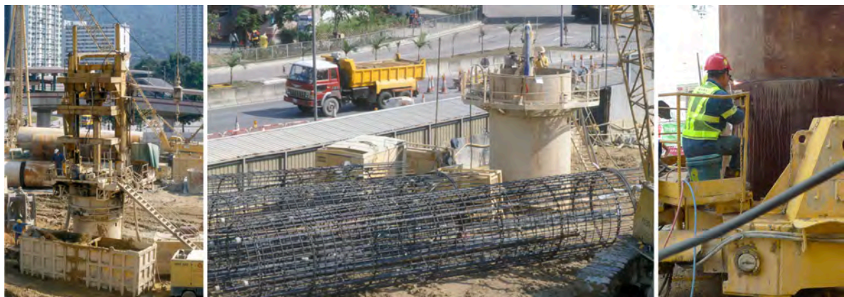
Figure D3.7: Large diameter bored pile work. Tai Wai
