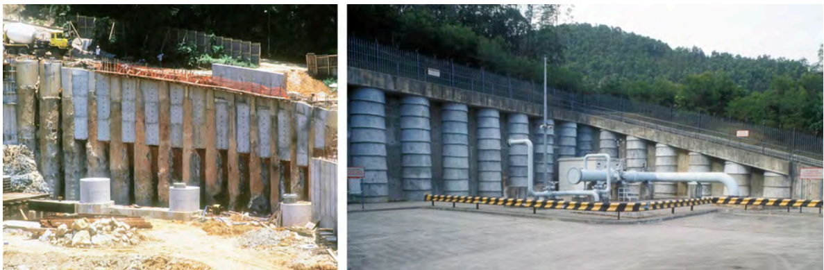
Figure D2.5: Bored contiguous pile walls.
