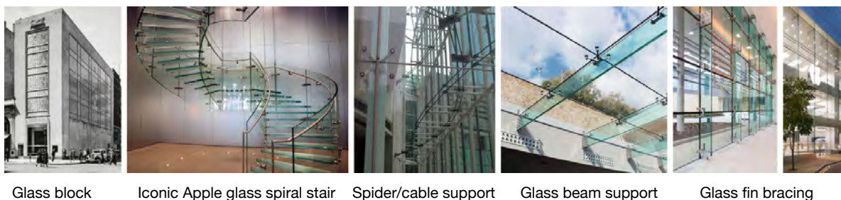
Figure C2.7: Structural Glass. Examples.
