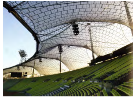
Figure A1.4b: A cable-net roof membrane
