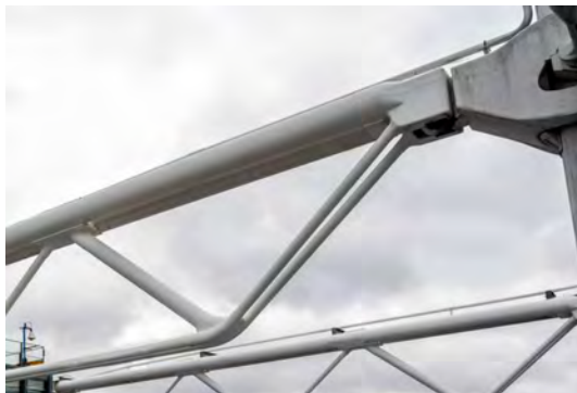
Figure E1.2: Types of connections: fixed joint (left) and hinge joint (right)
