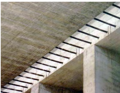
From top clockwise. Aerial view. The apparent visual thinness of the canopy contrasted with the monumental scale porticos that support it. View of portico with green tile surfaces. View of exposed steel cables at the edges of the slab.
