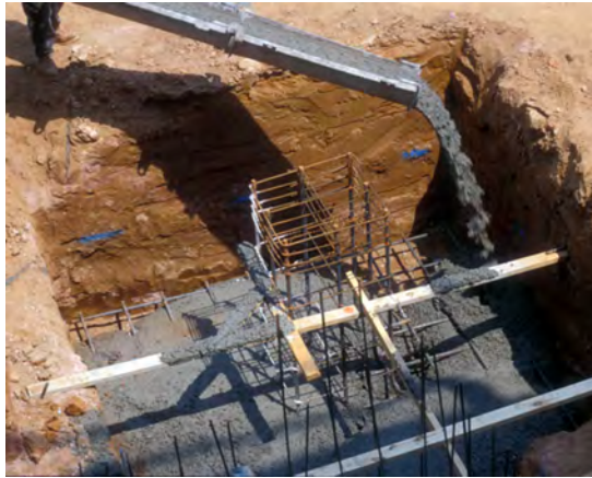
Figure D3.4: Spread Footings. Building Construction Illustrated , Francis D.K. Ching.
