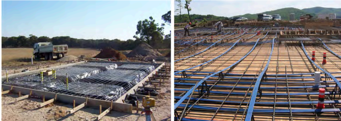
Figure D3.2: Ribbed and PT slab-on-grade
