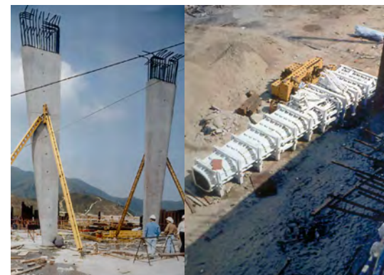
Above right: Specially designed steel forms for the tapered columns.
