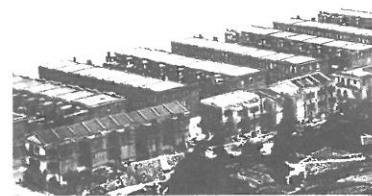
Buildings built to Building Ordinance 1903 in Shaukiwan, 1933. (Taken from Urban Council, 'The Hong Kong Album', Tat Shing Offset Printing Co Ltd., 1982.)
