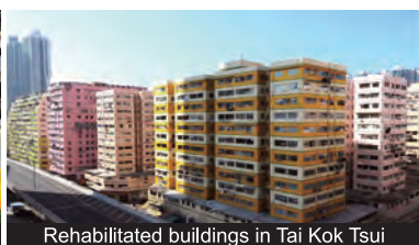
Rehabilitated buildings in Tai Kok Tsui
