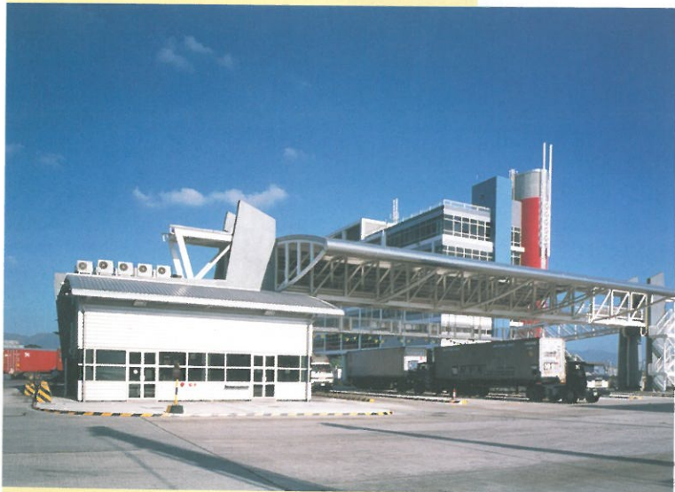
T8 West Entry Gatehouse
